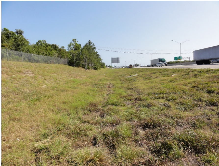
Photo 3. Roadside swale, on the east side of I-95 facing south
